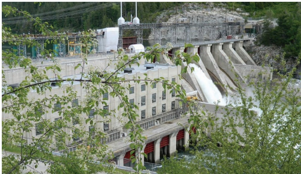
Brilliant Dam and Generating Station.
