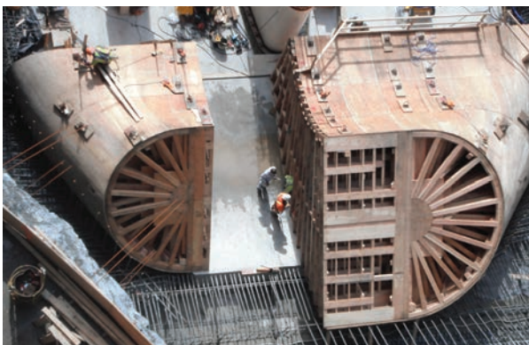
Wooden draft tube forms placed at the base of the Waneta Expansion Project powerhouse.
