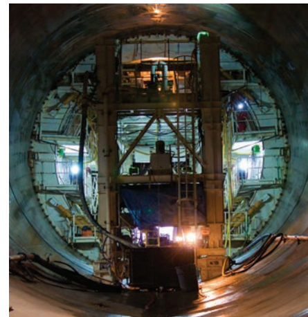
Travelling tunnel form placing the concrete lining inside one of the 10.5 metre diameter intake tunnels.
