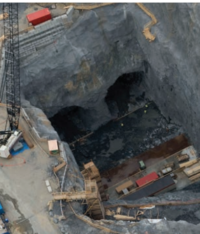
The intake tunnels at the Waneta Expansion will deliver water to the future powerhouse.
