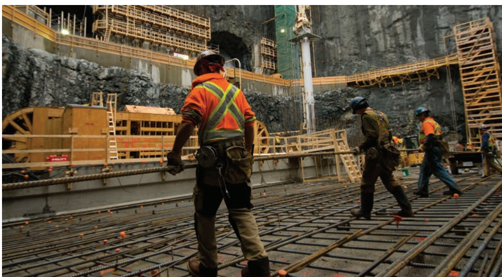
Workers safely navigating their steps as they prepare for a major concrete placement at the base of the powerhouse.
