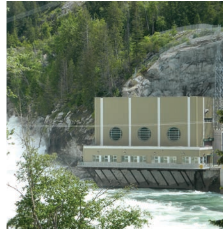
Brilliant Expansion Generating Station.
